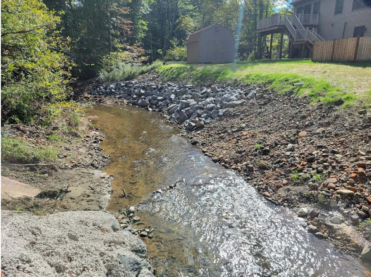
**Figure 7.** Gardner Creek at site GC03. Note the recent bank stabilization and grading completed during summer 2021 after heavy rainfall negatively impacted the area.
