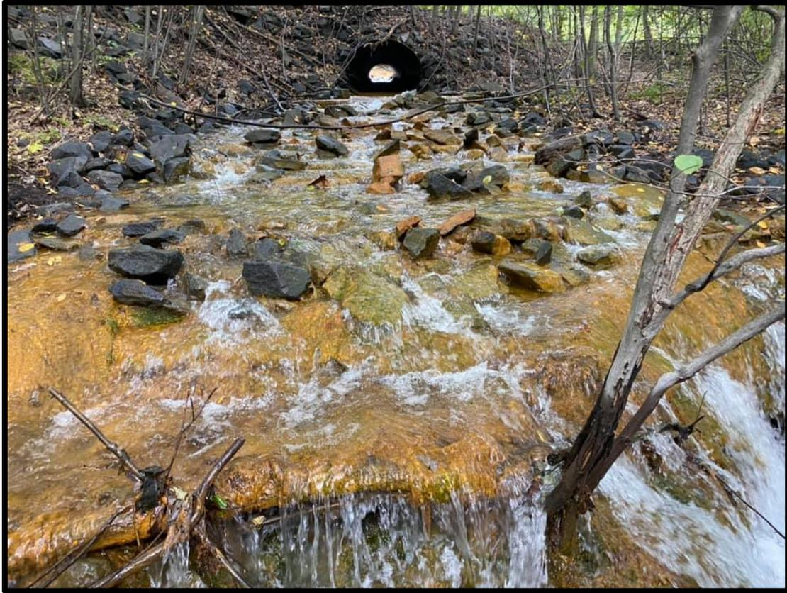
*Figure 24. Looking upstream on the Packer Air Shaft AMD discharge thru the squashed corrugated metal pipe culvert*
