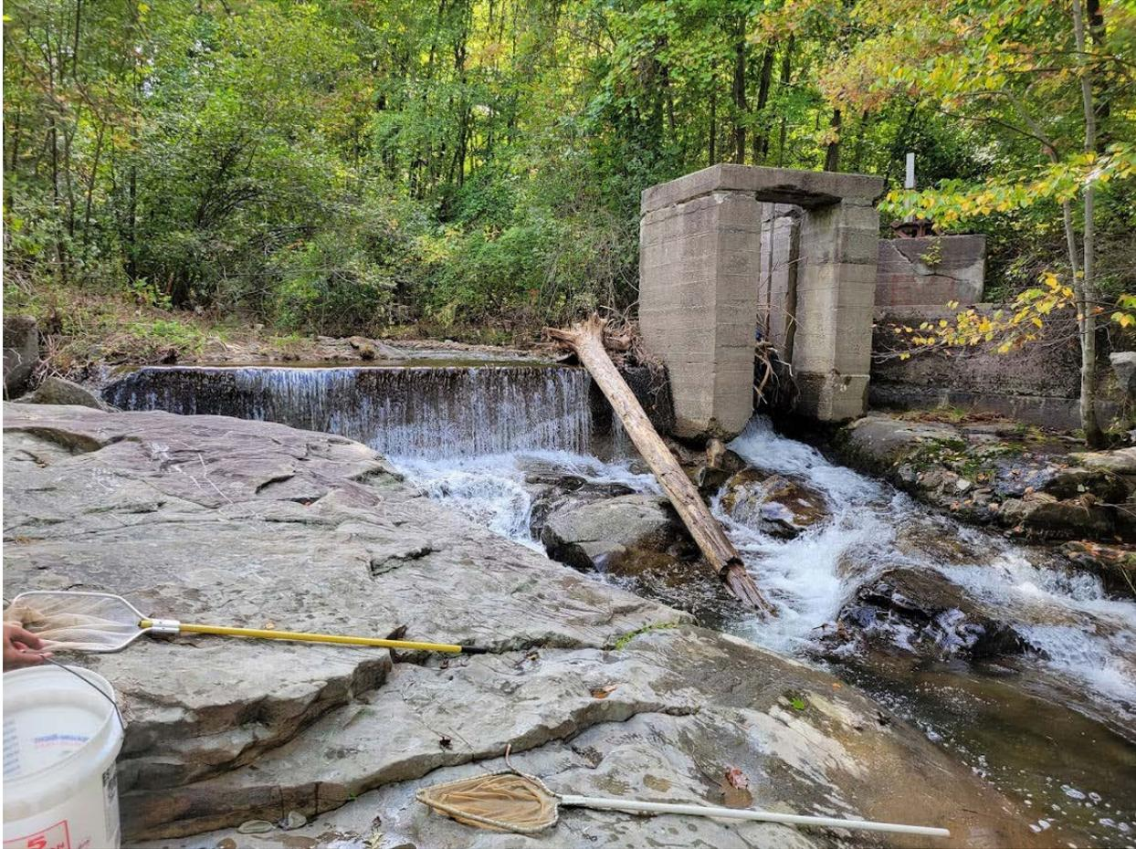
**Figure 10.** Old water withdrawal structure and dam at site MC04 downstream of the railroad tunnel on Old Pittston Blvd posing a barrier to aquatic organism passage. Trout were documented upstream and downstream of this structure.
