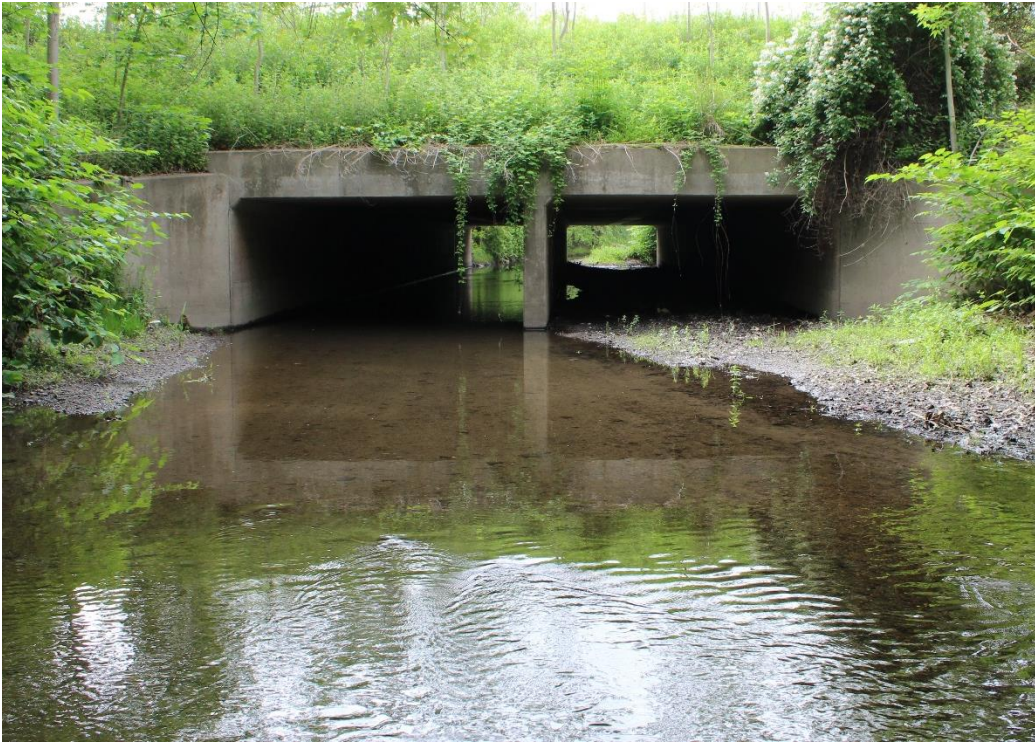
Figure 7: LR1 Upstream (Photo 2)
