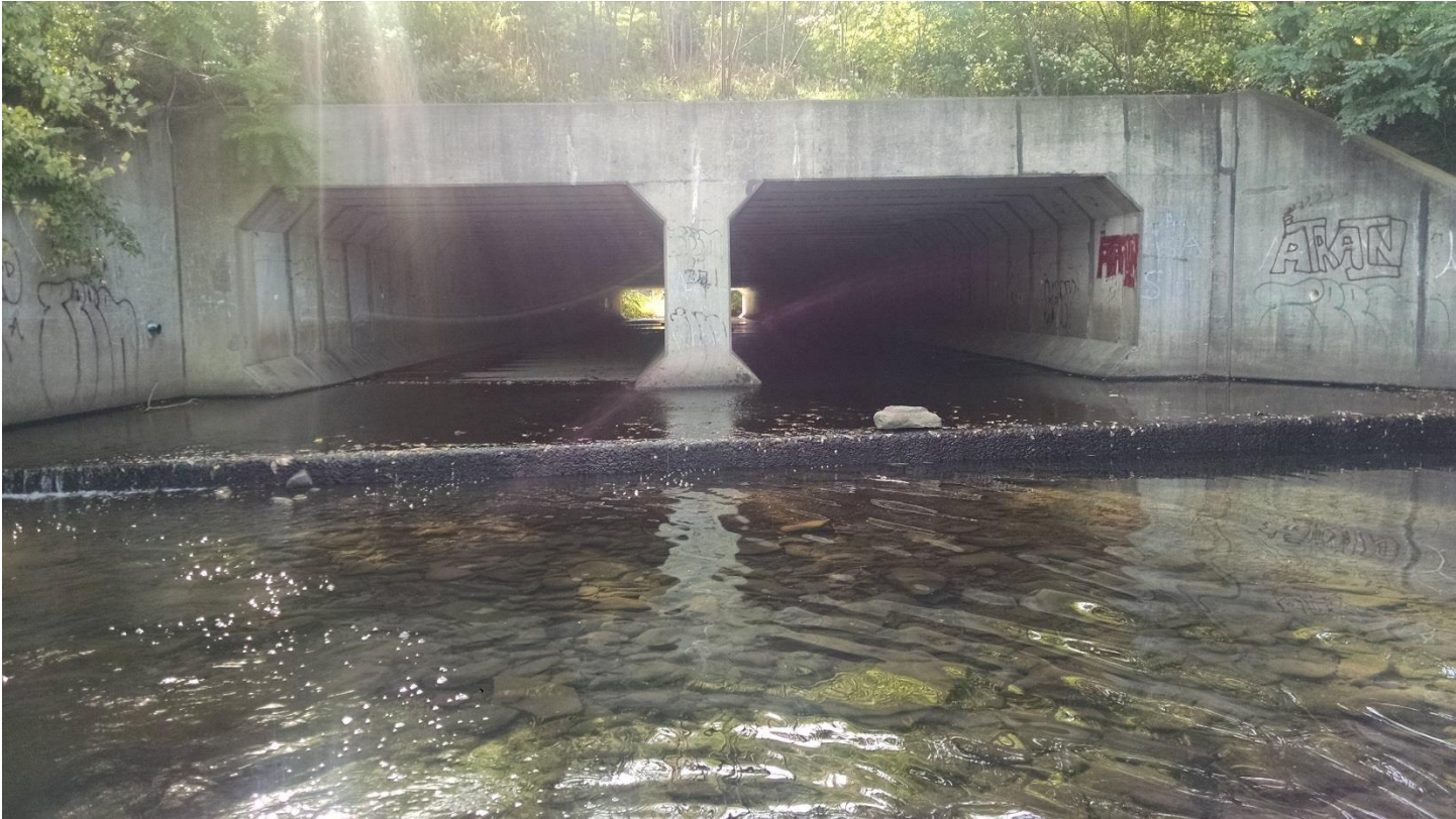
Figure 63: Culvert #3 Outlet (Photo 59)
