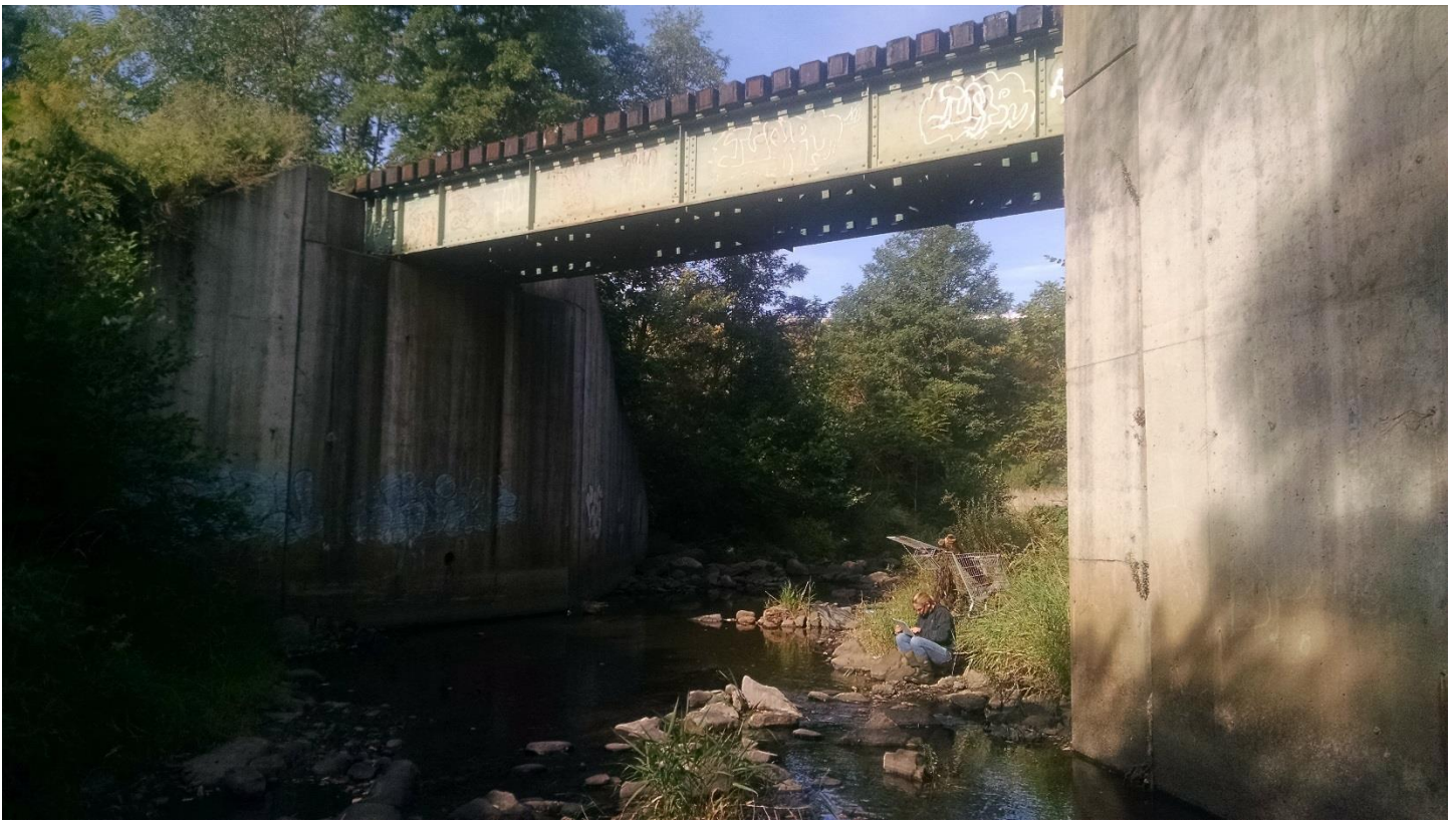
Figure 64: Train Crossing Inlet (Photo 60)
