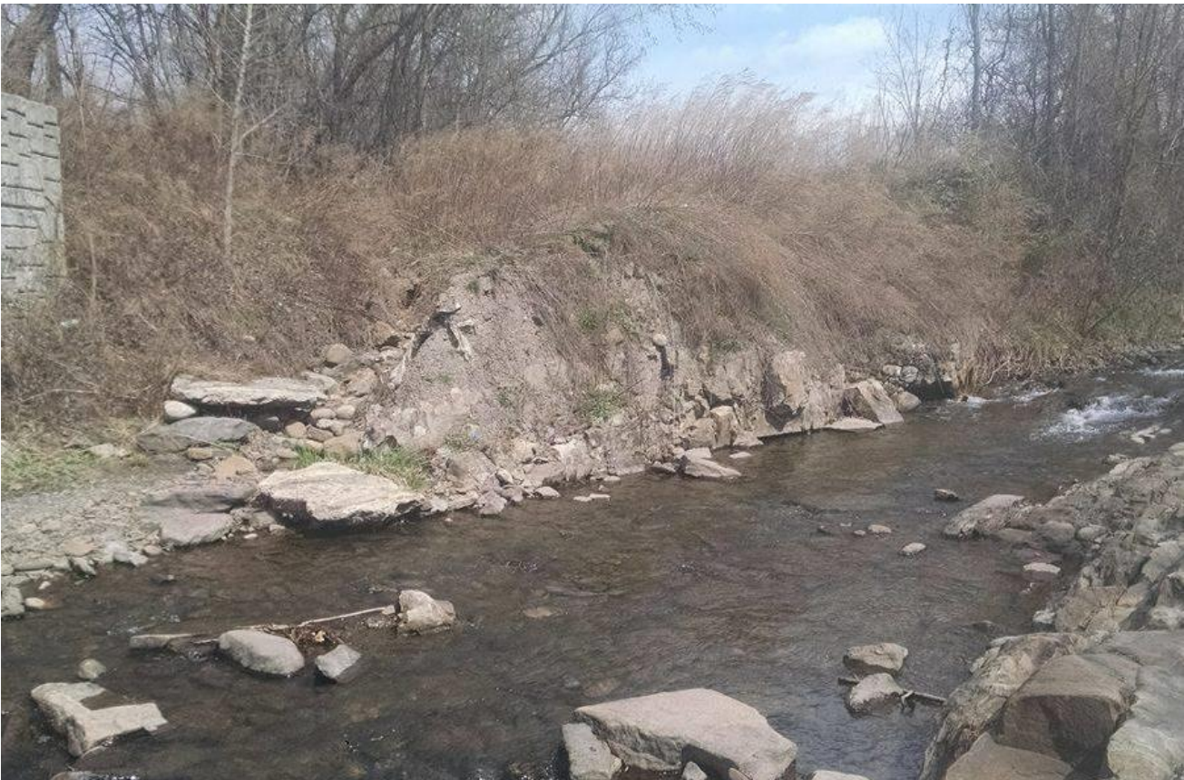
Figure 16: Erosion near LR4 (Photo 11)
