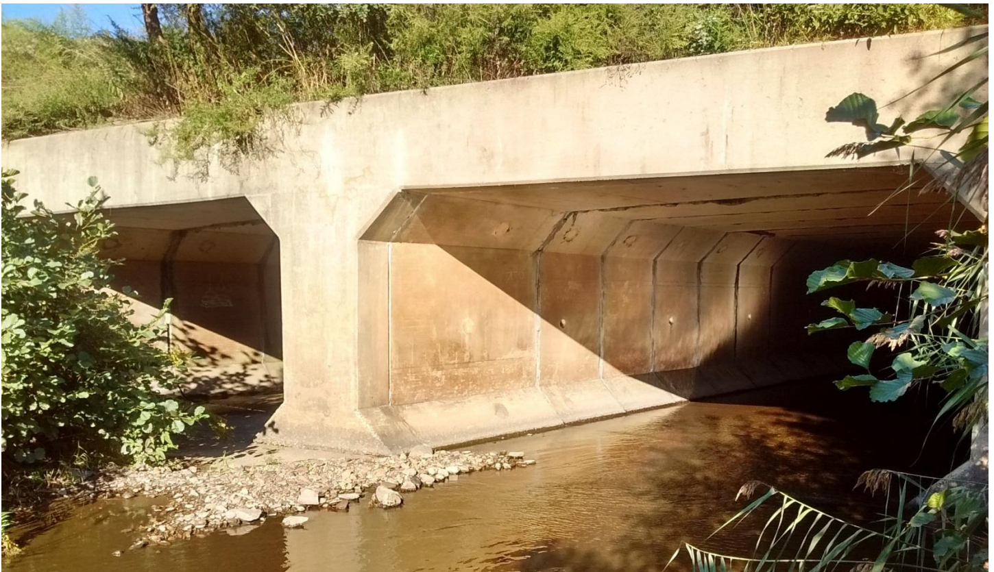
Figure 60: Culvert #2 Inlet (Photo 56)
