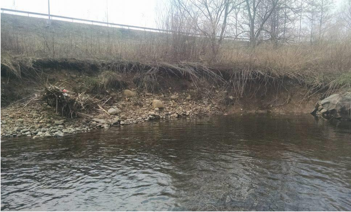
Figure 17: Erosion Near LR4 (Photo 12)
