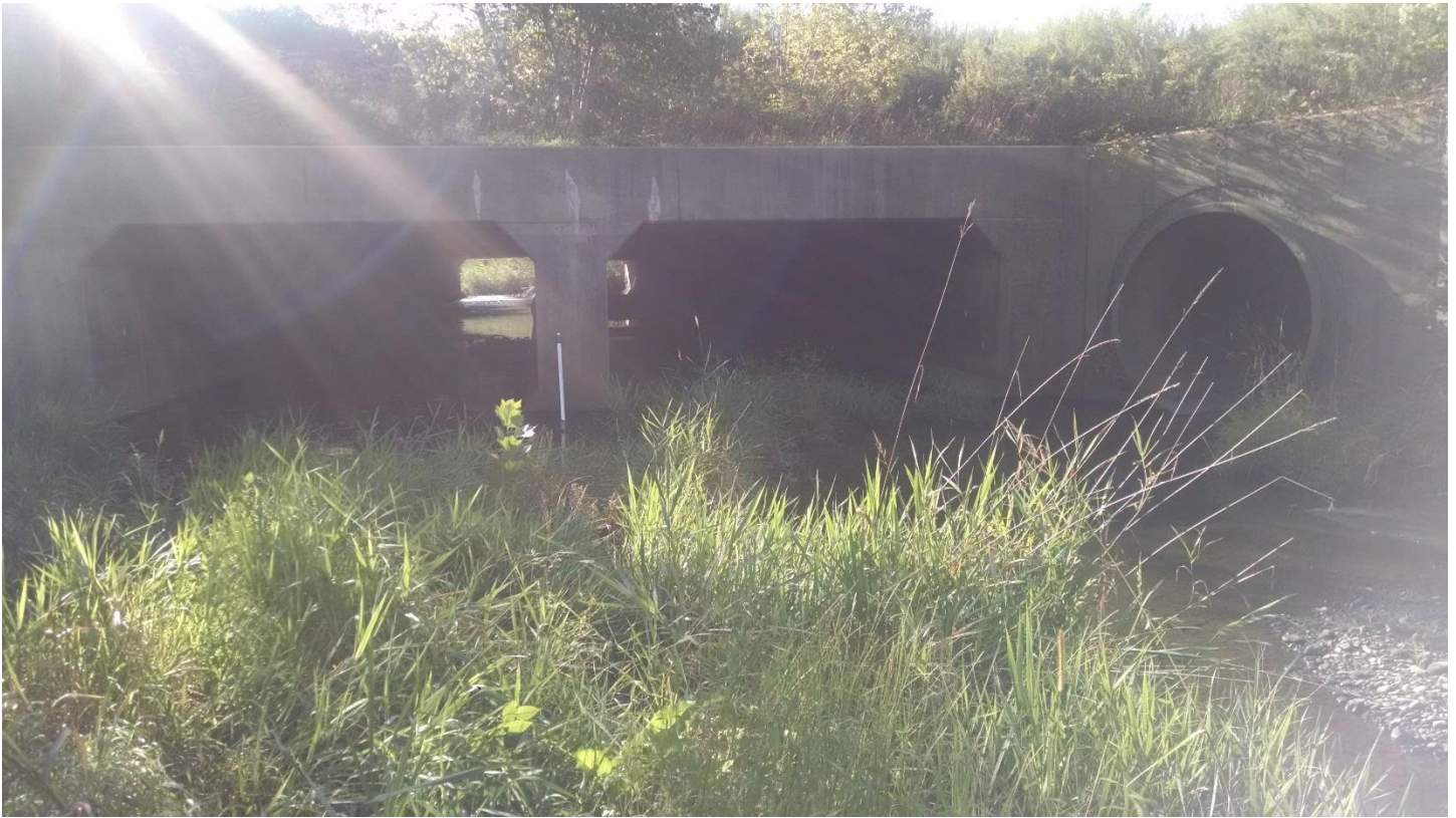
Figure 61: Culvert #2 Outlet (Photo 57)
