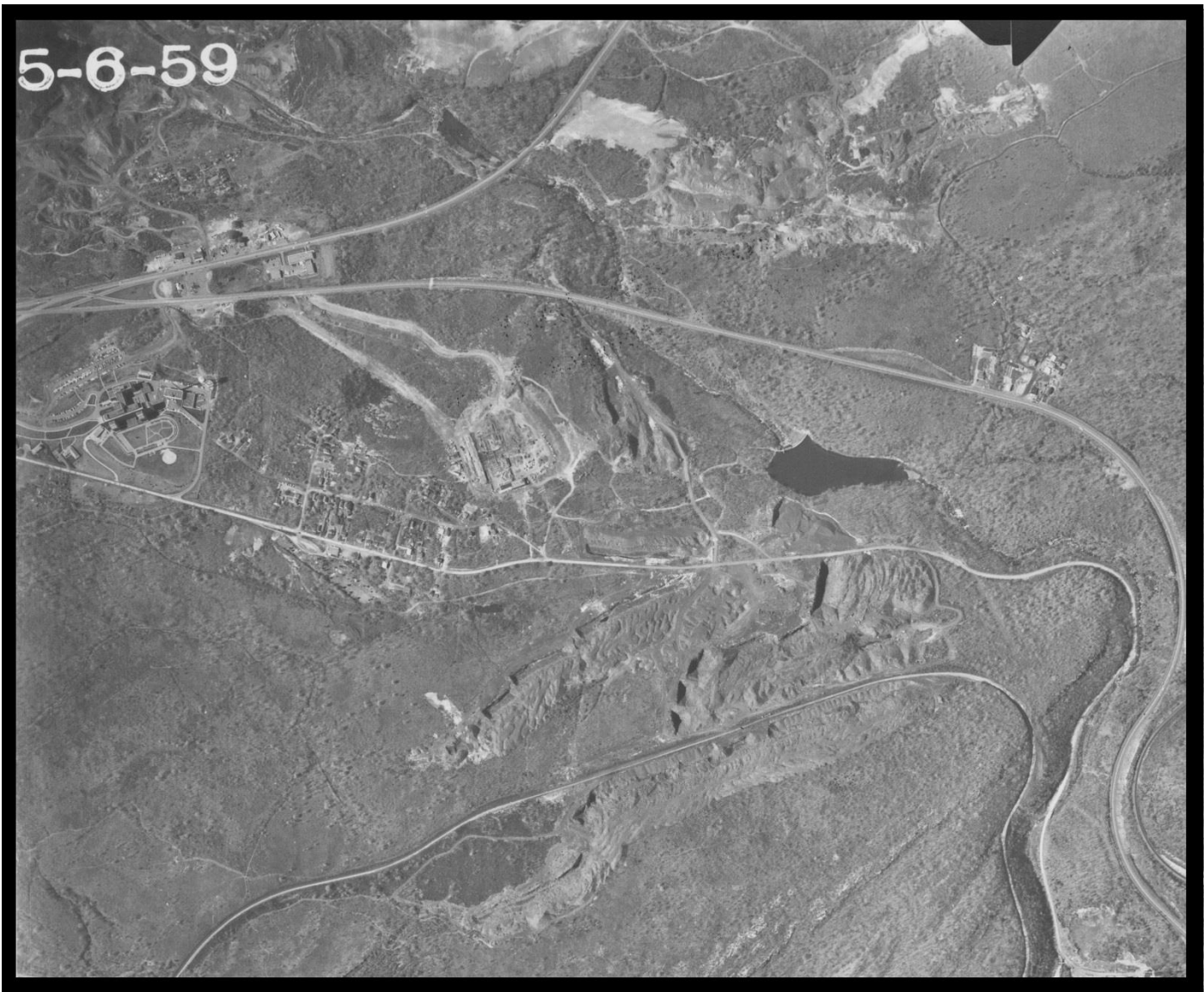
Figure 68: Laurel Run #2 Dam 1959 (Photo 55)
