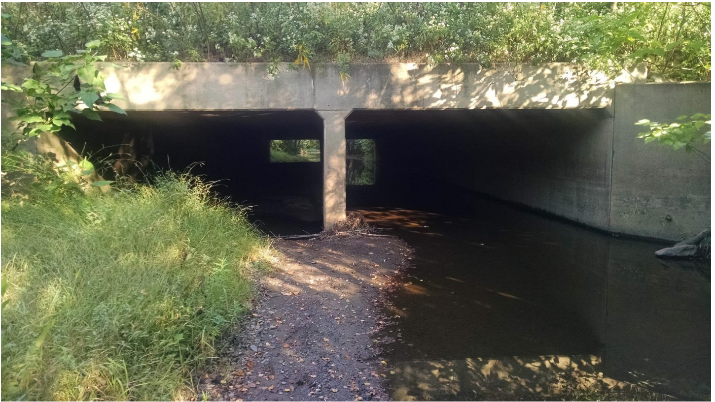
Figure 58: Culvert #1 Inlet (Photo 54)
