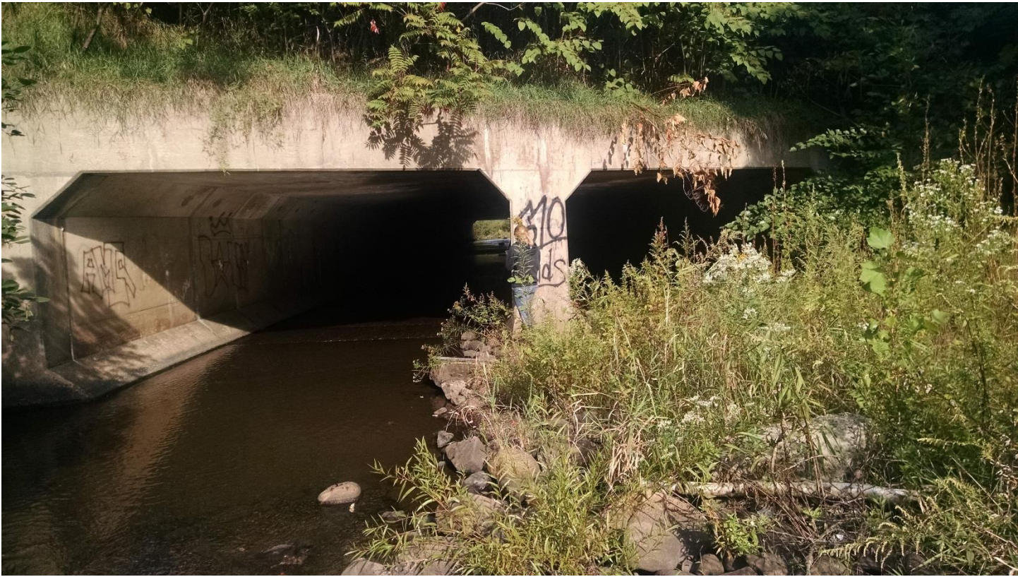
Figure 62: Culvert #3 Inlet (Photo 58)
