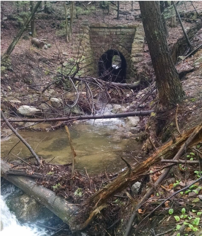
Figure 32: LR_UNT_WB2 Upstream (Photo 28)
