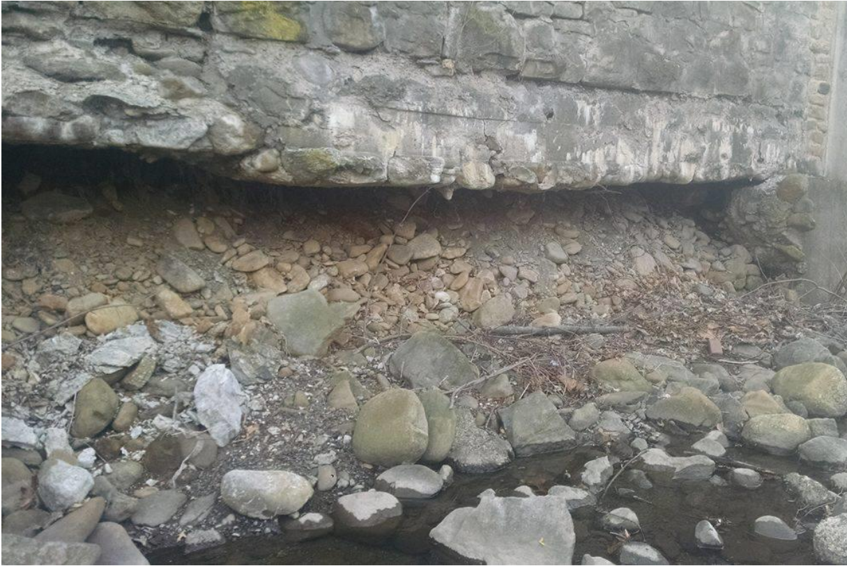
Figure 18: Flood Wall Undercutting (Photo 13)
