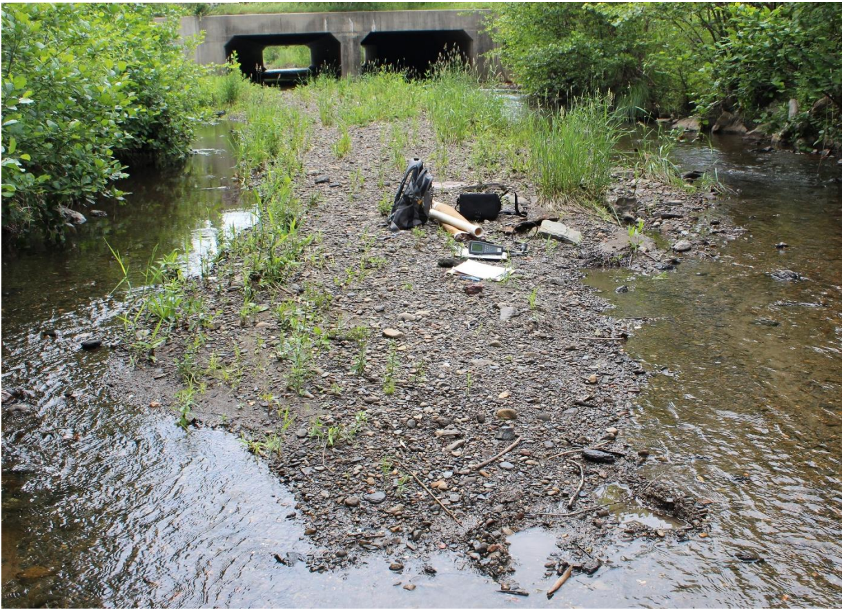
Figure 9: LR2 Upstream (Photo 4)
