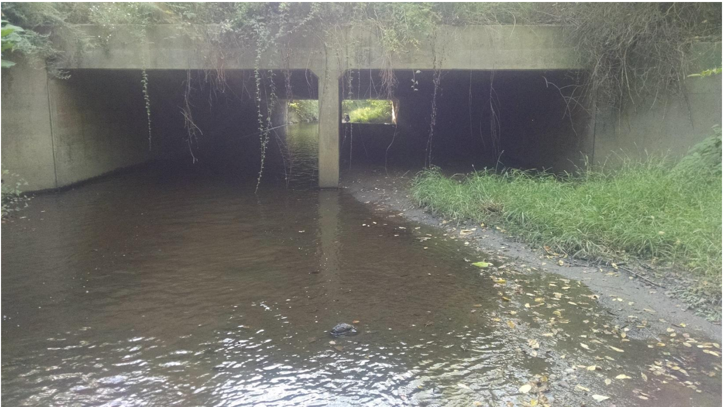
Figure 59: Culvert #1 Outlet (Photo 55)
