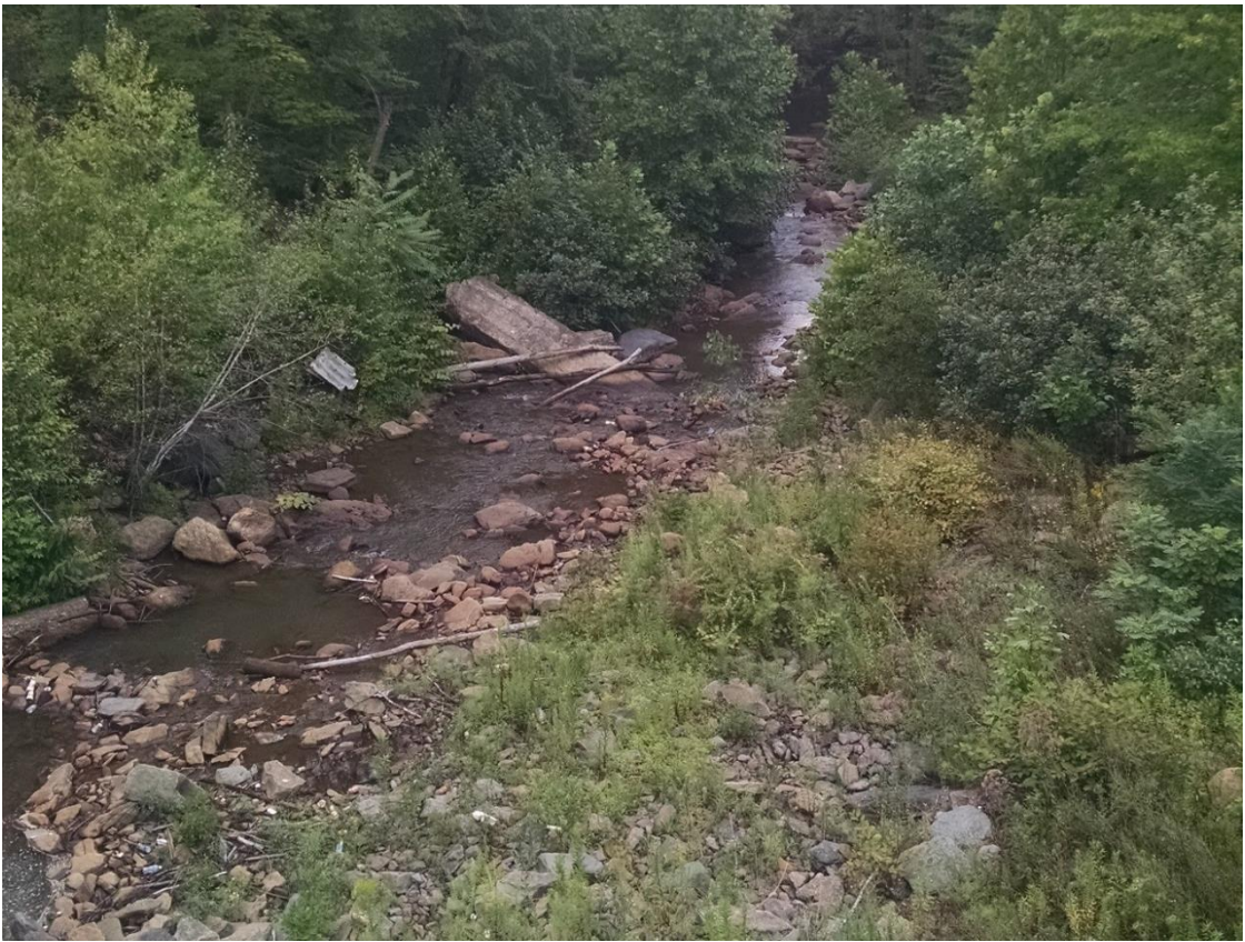
Figure 21: LR6 Downstream - AMD Staining from seep (Photo 16)
