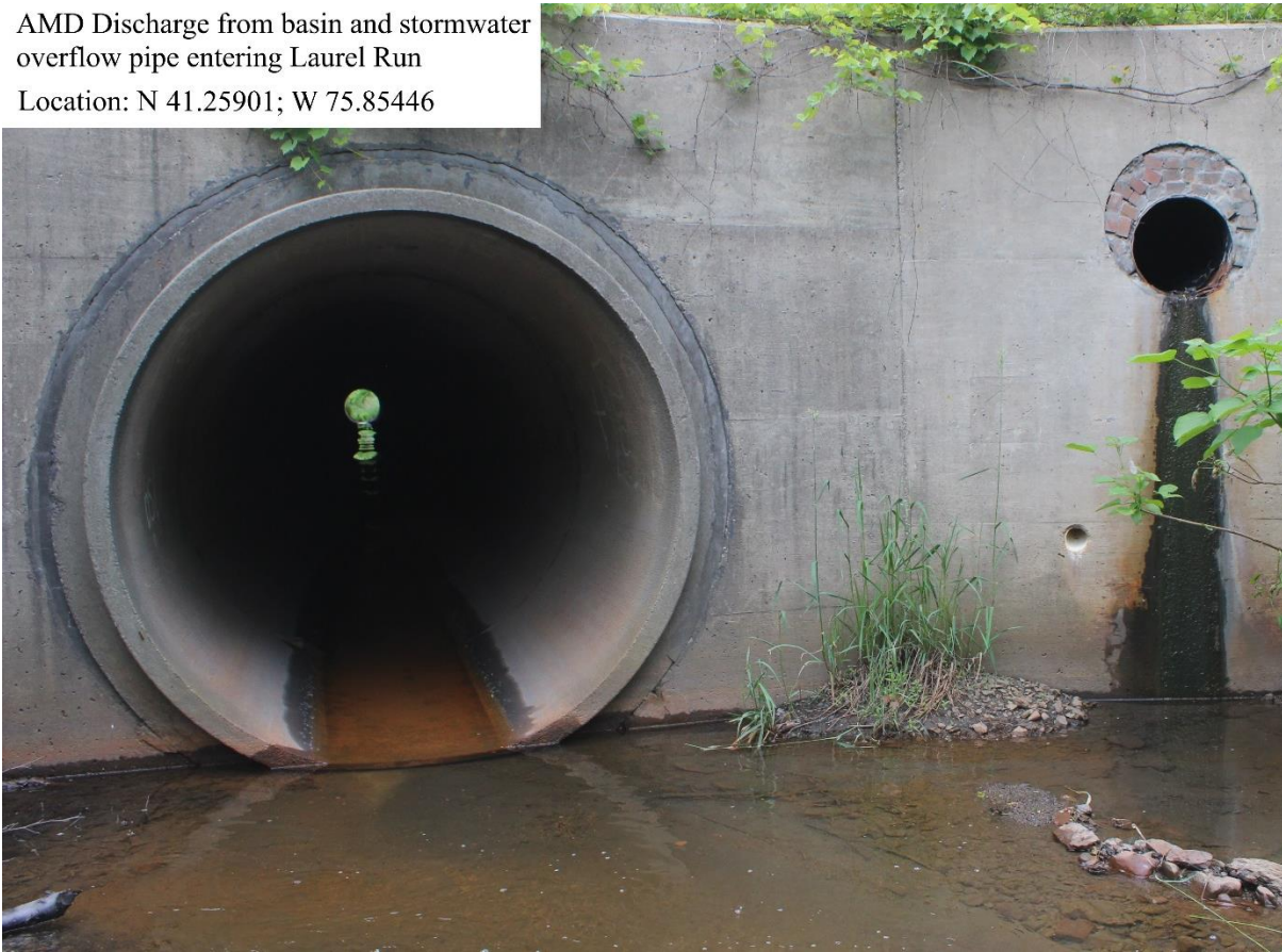
Figure 11: LR2 AMD seep discharge from small basin (Photo 6)
