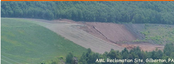
AML Reclamation Site, Gilberton, PA
