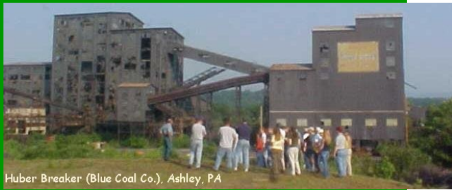
Huber Breaker (Blue Coal Co.), Ashley, PA
