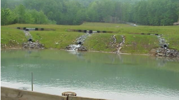
Oneida #1 AMD Passive Treatment System (Oxic Limestone Drain), Eagle Rock, PA
